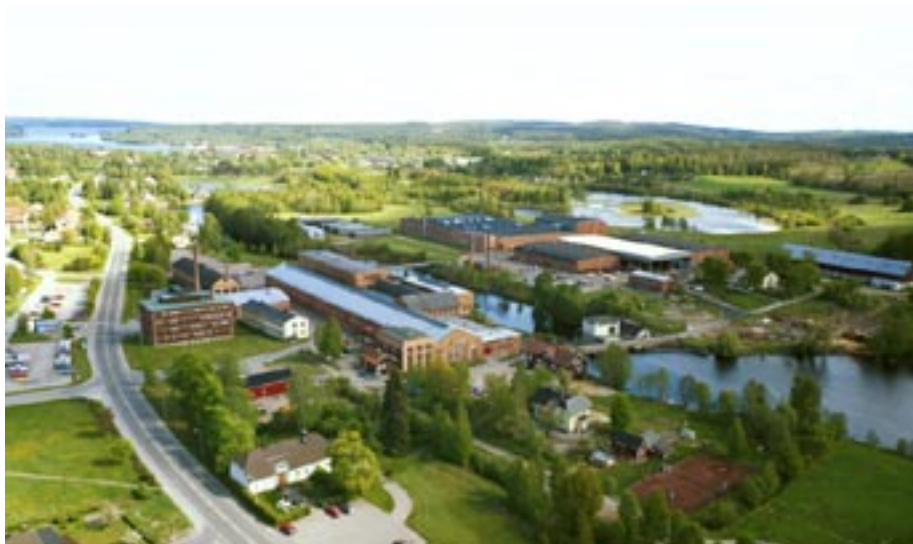
The Morgårdshammar plant in Smedjebacken, Sweden
